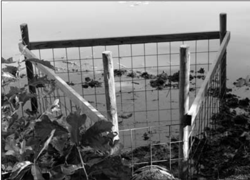
Figure 29 A small beaver “deceiver” built by Skip Lisle to protect a roadside culvert. Lasting upward of fifteen to twenty years, these devices are practical and economical, not to mention humane.
