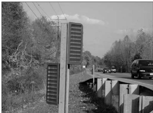
**Figure 49** *The roadside reflector (Streiter-Lite®) reflects headlights as a series of light beams (an “optical fence”) to keep deer from crossing in the path of oncoming vehicles. This and other technologies to help prevent deer-vehicle accidents are important in addressing this growing issue.*
