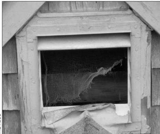
**Figure 70** The flimsy insect screen has been pushed aside as a raccoon has moved into this attic. Eviction with a one-way door and replacement of the screen with material sturdy enough to prevent another intrusion is called for here, not trapping.
